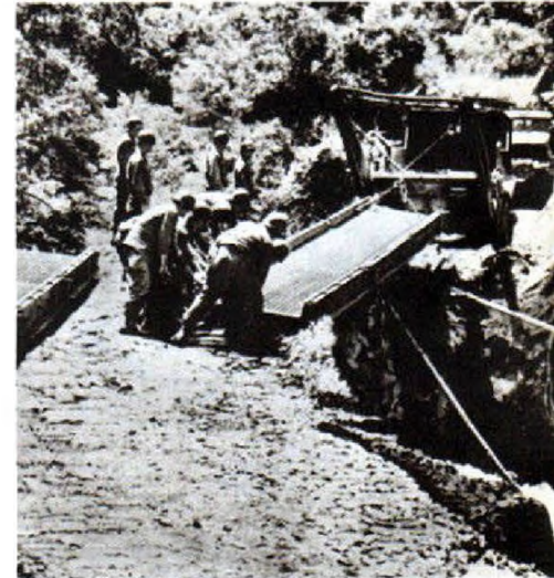
BUILDING BRIDGES IN A HURRY. For most of the material of defense, steel is essential. And because of its constantly expanding production capacity, United States Steel is able to contribute more and more of this vital metal to help safeguard America's security.
